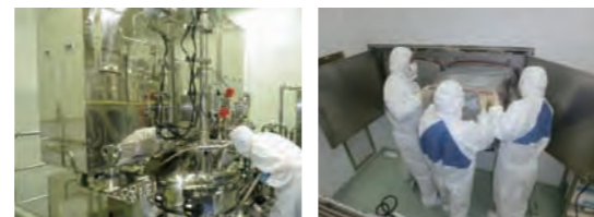
Exchange of HEPA filter Bag in-Bag out method
