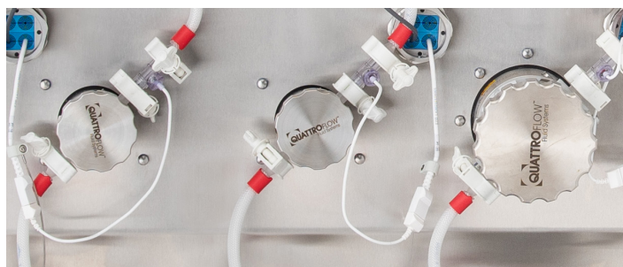
Figure 5. Three positive displacement pumps.
